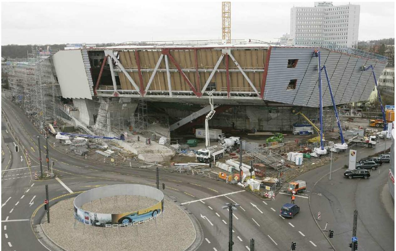
has currently reached a weight of 12,000 tons. This is lowered carefully from the scaffold towers into the steel-reinforced concrete supports. The weight after completion, that is after installing all extension and traffic loads, will grow to an incredible 35,000 tons. The forces acting on the supports are measured and set to nominal values.
